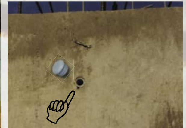
Concreted hexagon stop end sleeves
